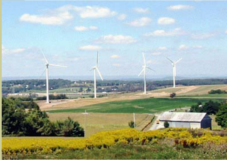
Turbines at the Somerset, Pa AML site
